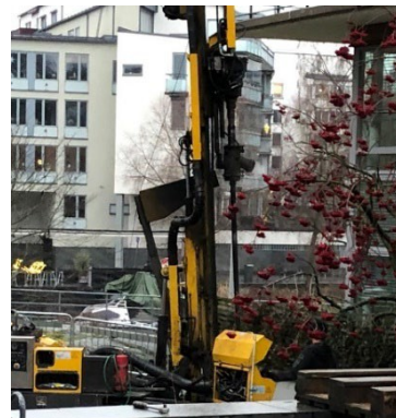
Borrning - Installation utmed Sickla Kanalgrata
